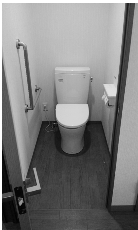
Fig. 2. Appearance of toilet room.
